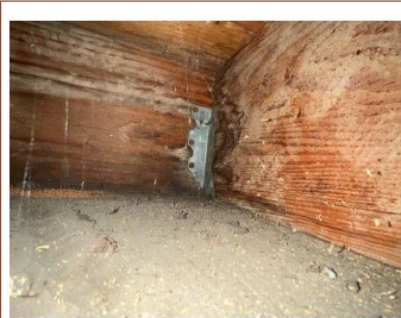
Underside of landing substrate and framing show signs of water intrusion
