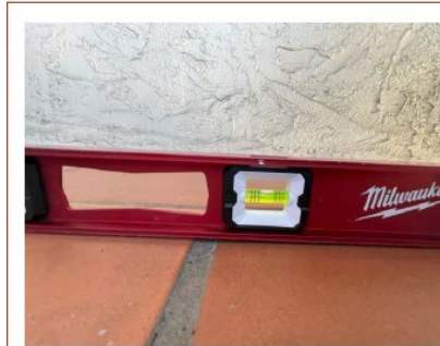
Landing surface is not sloped to encourage drainage
